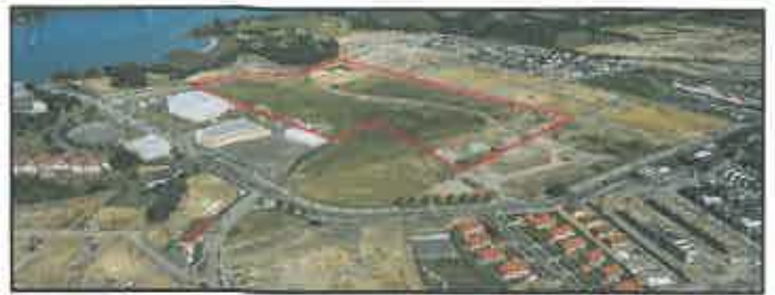
Stage Two development area
